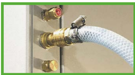
Pressed air connection for automatic cleaning
